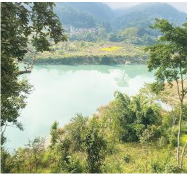
PHOTO: TRN River dam on Marsyangdi river in Anbukhaireni Rural Municipality-4, Tanahun.
