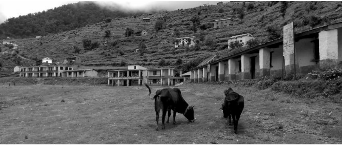
The transformed school in Mumbra village of Sanni-Triveni Rural Municipality, Kalikot, after fencing off the open area.
